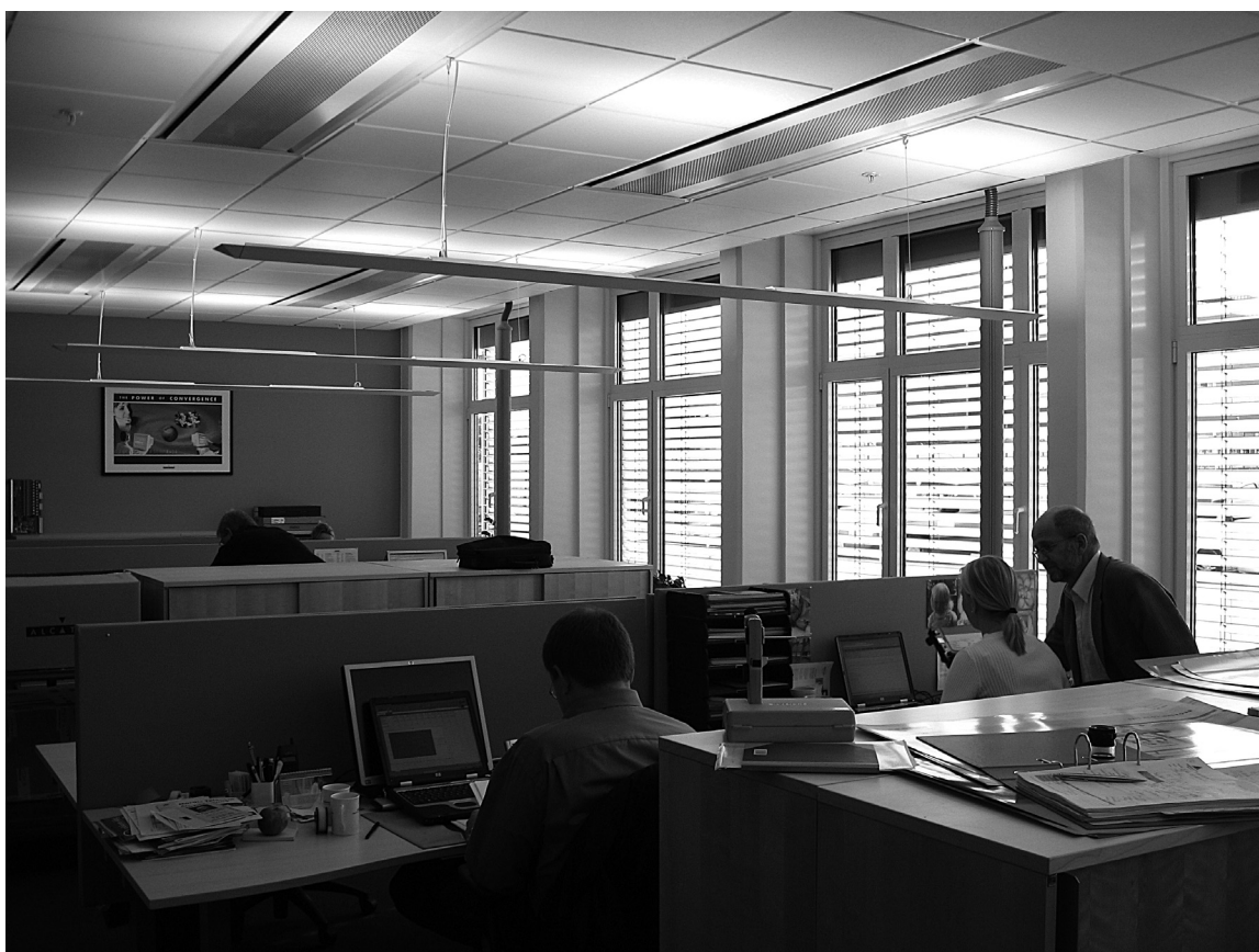
Figure 3. In the office landscape the luminaires were positioned parallel to the length of the tables providing only indirect lighting. Notes. Luminance from the ceiling was 600–800 \text{cd/m}^2 .
